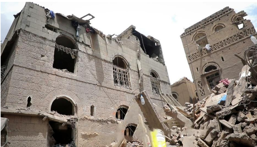
Traditional houses in Old Sana'a damaged by Israeli airstrikes, September 10, 2025
