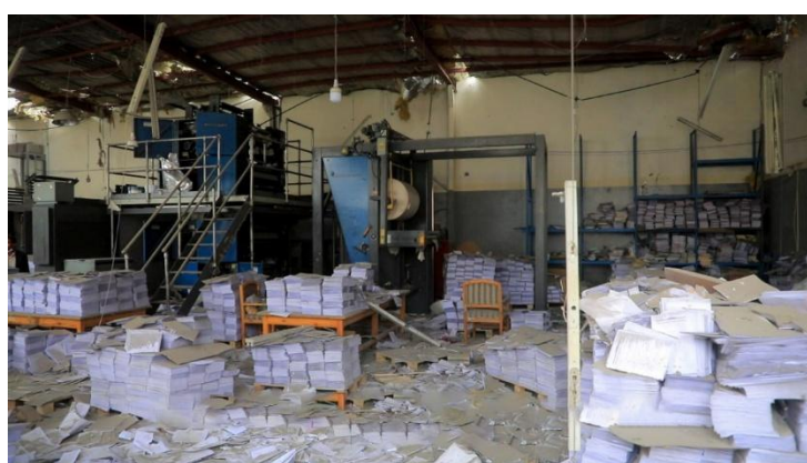
Some of the damage inflicted on the printing presses of "26 September" newspaper following Israeli airstrikes, September 10, 2025
